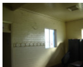
poplar oval pavilion interior with coat hooks jun07 jmb
