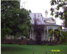
23360 School Master s Residence Former 59 Bell St Penshurst 0916
