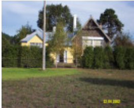
23363 State School 486 Former 67 Watton St Penshurst 0819
