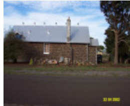
23363 State School 486 Former 67 Watton St Penshurst 0822
