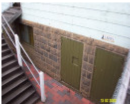
23379 Grandstand Racecourse Penshurst bar toilets 1544
