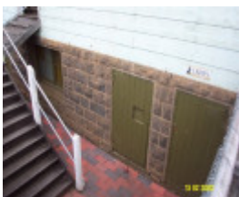
23379 Grandstand Racecourse Penshurst bar toilets 1544
