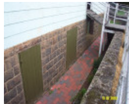
23379 Grandstand Racecourse Penshurst bar toilets 1543
