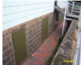
23379 Grandstand Racecourse Penshurst bar toilets 1543
