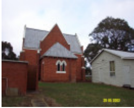
23385 St Andrews Uniting Ch Glenthompson rear 1042
