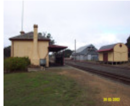
23389 Railway Station Complex Glenthompson 1060
