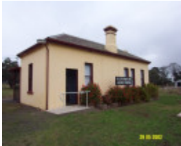
23389 Railway Station Complex Glenthompson 1057
