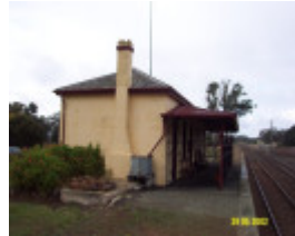
23389 Railway Station Complex Glenthompson 1058
