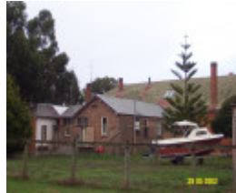
23394 Mac s Hotel Station St Glenthompson rear 1097
