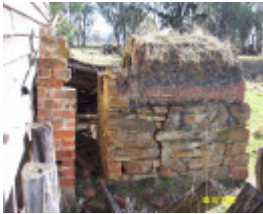
23404 Ruined House Mirranatwa oven 1139
