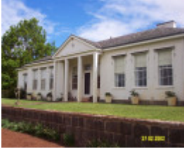
23413 Nareeb Nareeb facade 1672
