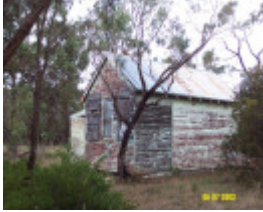
23416 Former School Mooralla 1176
