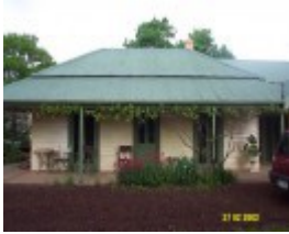
23418 Stirling Homestead Glenthompson facade 1681
