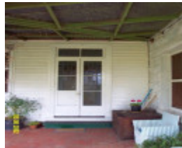
23419 Lovatdale Glenthompson detail of verandah 1234
