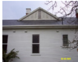
23419 Lovatdale Glenthompson west elevation 1238
