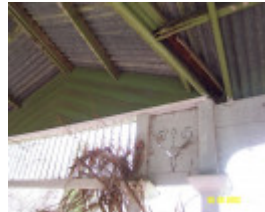
23419 Lovatdale Glenthompson detail of verandah 1236
