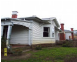
23419 Lovatdale Glenthompson west elevation 1229
