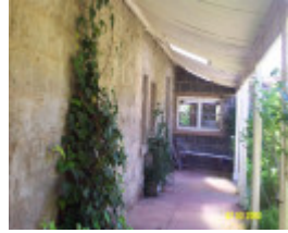
23426 Woodhouse side verandah 1734
