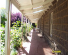
23426 Woodhouse front verandah 1732
