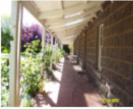
23426 Woodhouse front verandah 1732
