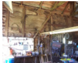
23426 Woodhouse stables slab wall 1741
