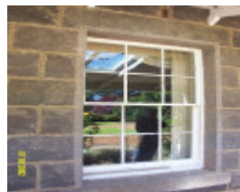
23426 Woodhouse facade window 1726
