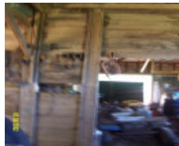
23426 Woodhouse stables slab wall 1742
