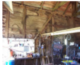
23426 Woodhouse stables slab wall 1741
