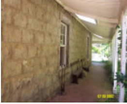
23426 Woodhouse side verandah 1731
