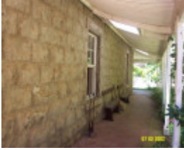
23426 Woodhouse side verandah 1731
