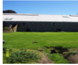
23426 Woodhouse woolshed drain 1751
