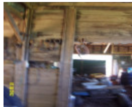
23426 Woodhouse stables slab wall 1742
