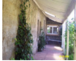
23426 Woodhouse side verandah 1734
