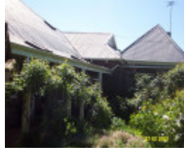
23426 Woodhouse side verandah kitchen 1735
