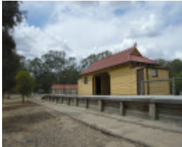
KOONDROOK TRAM COMPLEX SOHE 2008
