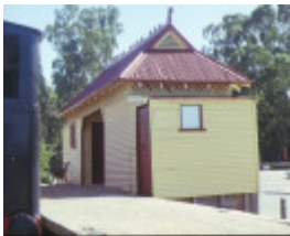
1 tram station koondrook tram station side view jan1990
