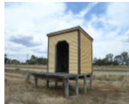
KOONDROOK TRAM COMPLEX SOHE 2008
