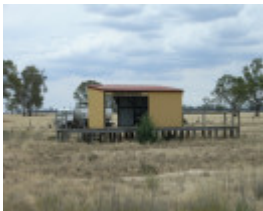
KOONDROOK TRAM COMPLEX SOHE 2008
