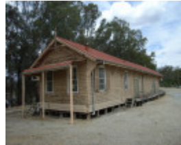
KOONDROOK TRAM COMPLEX SOHE 2008
