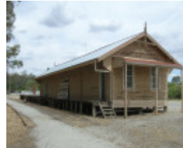
KOONDROOK TRAM COMPLEX SOHE 2008
