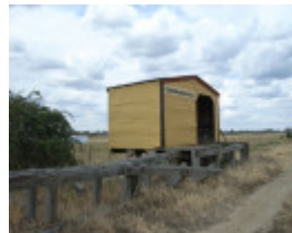
KOONDROOK TRAM COMPLEX SOHE 2008
