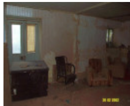
23435 Skene Homestead Strathkellar 1858 cellar 1590
