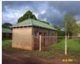
23435 Skene Homestead Strathkellar generator shed
