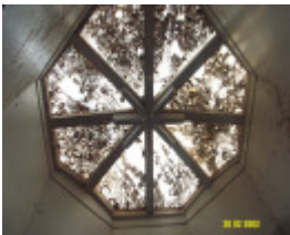
23435 Skene Homestead Strathkellar 1858 skylight 1613
