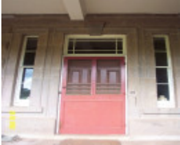
23435 Skene Homestead Strathkellar 1858 front door 1556
