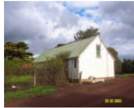
23435 Skene Homestead Strathkellar outbuilding 1578
