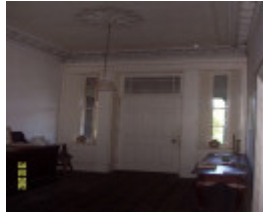
23435 Skene Homestead Strathkellar 1858 front door 1582
