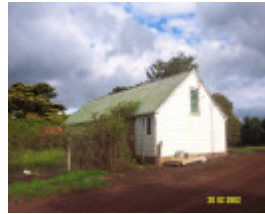
23435 Skene Homestead Strathkellar outbuilding 1578
