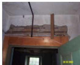
23435 Skene Homestead Strathkellar 1858 cellar 1601
