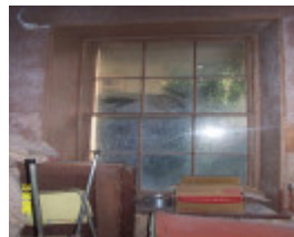
23435 Skene Homestead Strathkellar 1858 cellar 1594
