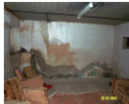
23435 Skene Homestead Strathkellar 1858 cellar 1589
