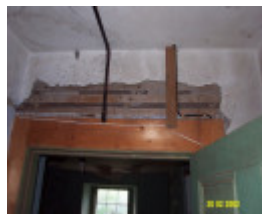
23435 Skene Homestead Strathkellar 1858 cellar 1601
