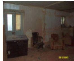
23435 Skene Homestead Strathkellar 1858 cellar 1590
