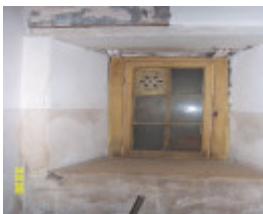
23435 Skene Homestead Strathkellar 1858 cellar 1598
