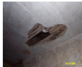
23435 Skene Homestead Strathkellar 1858 cellar 1595
