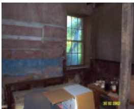
23435 Skene Homestead Strathkellar 1858 cellar 1593
