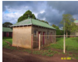
23435 Skene Homestead Strathkellar generator shed
