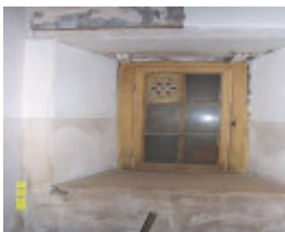
23435 Skene Homestead Strathkellar 1858 cellar 1598
