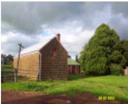
23435 Skene Homestead Strathkellar generator shed 1575
