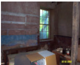
23435 Skene Homestead Strathkellar 1858 cellar 1593
