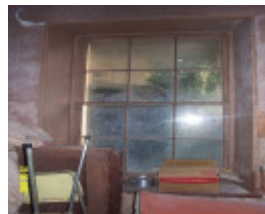
23435 Skene Homestead Strathkellar 1858 cellar 1594
