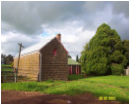
23435 Skene Homestead Strathkellar generator shed 1575
