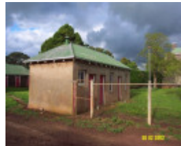
23435 Skene Homestead Strathkellar generator shed
