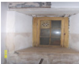
23435 Skene Homestead Strathkellar 1858 cellar 1598
