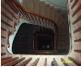
23435 Skene Homestead Strathkellar 1858 staircase 1615
