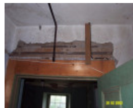
23435 Skene Homestead Strathkellar 1858 cellar 1601
