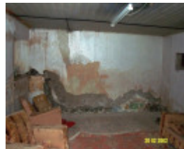
23435 Skene Homestead Strathkellar 1858 cellar 1589
