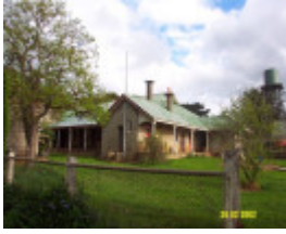
23435 Skene Homestead Strathkellar utility shed 1574
