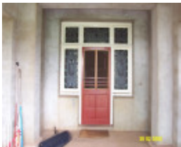
23435 Skene Homestead Strathkellar 1923 front door 1567
