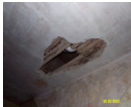
23435 Skene Homestead Strathkellar 1858 cellar 1595
