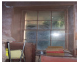
23435 Skene Homestead Strathkellar 1858 cellar 1594
