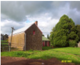
23435 Skene Homestead Strathkellar generator shed 1575
