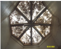
23435 Skene Homestead Strathkellar 1858 skylight 1613
