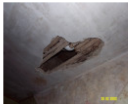
23435 Skene Homestead Strathkellar 1858 cellar 1595
