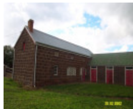
23435 Skene Homestead Strathkellar stables 1573
