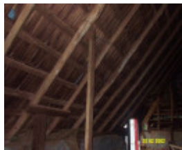
23435 Skene Homestead Strathkellar woolshed poles shingles 1635
