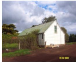
23435 Skene Homestead Strathkellar outbuilding 1578
