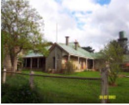
23435 Skene Homestead Strathkellar utility shed 1574
