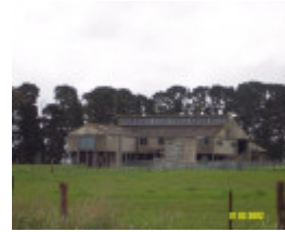
23441 Torbank Woolshed Tobermory Rd Penshurst 1715
