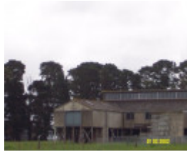
23441 Torbank Woolshed Tobermory Rd Penshurst 1714
