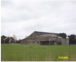
23441 Torbank Woolshed Tobermory Rd Penshurst 1713
