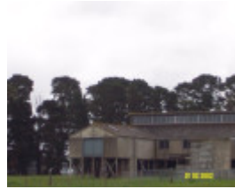
23441 Torbank Woolshed Tobermory Rd Penshurst 1714
