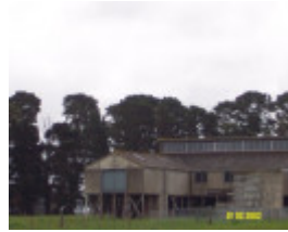
23441 Torbank Woolshed Tobermory Rd Penshurst 1714
