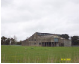
23441 Torbank Woolshed Tobermory Rd Penshurst 1713
