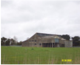
23441 Torbank Woolshed Tobermory Rd Penshurst 1713
