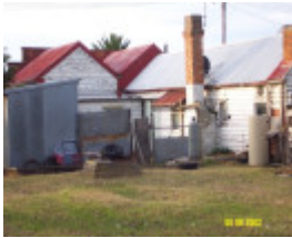
23454 Turners Store Glenthompson rear view 1105
