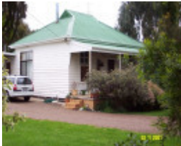
23477 Timber Cottage Cavendish 0117
