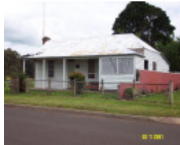
23477 Timber Cottage Cavendish 0118
