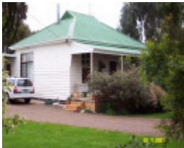
23477 Timber Cottage Cavendish 0117
