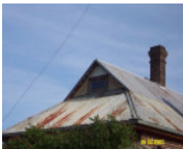
23480 Myrning Wootong Vale roof detail 2007
