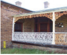
23480 Myrniong Wootong Vale verandah 1997
