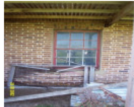
23480 Myrning Wootong Vale basement window 2003
