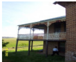
23480 Myrning Wootong Vale side verandah 2002
