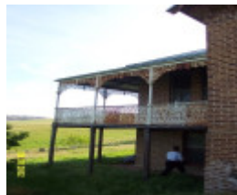
23480 Myrning Wootong Vale side verandah 2002
