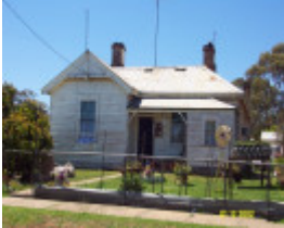
23481 Police station residence former Balmoral 2098
