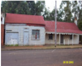
23483 Stewart s Store Residence Station St Glenthompson 1064
