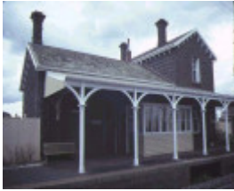
Source: Victorian Heritage Register. Taken 1984.
