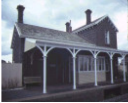
Source: Victorian Heritage Register. Taken 1984.
