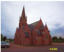
23498 St Michael s Lutheran Complex Tarrington church 0946
