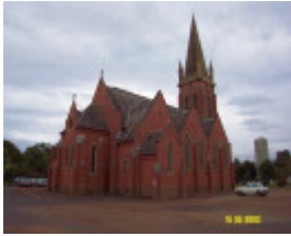
23498 St Michael s Lutheran Complex Tarrington church 0947
