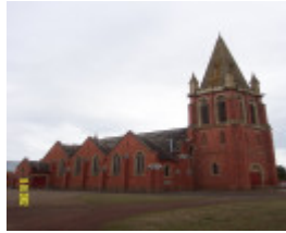
23498 St Michael s Lutheran Complex Tarrington church 0950
