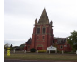
23498 St Michael s Lutheran Complex Tarrington church 0953
