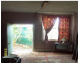
23499 Former School Gritjurk residence 2022
