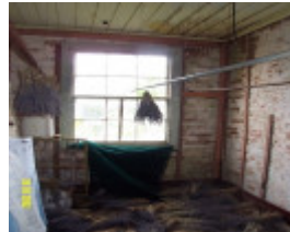
23499 Former School Gritjurk residence 2025
