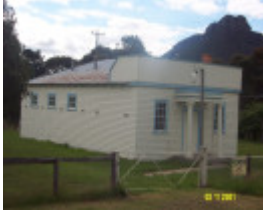
23501 Masonic Hall Former Dunkeld 0158
