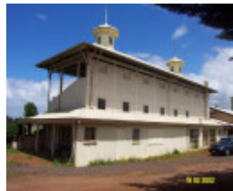
23522 Hamilton Racecourse Grandstand old rear 1845
