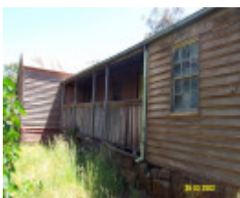
23526 Hillview Nareen verandah 1965
