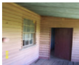
23526 Hillview Nareen verandah 1968
