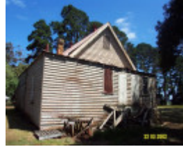
23541 Strathkellar Mechanics Institute 1907
