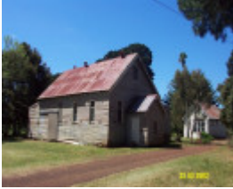
23541 Strathkellar Mechanics Institute 1904
