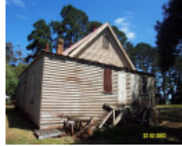
23541 Strathkellar Mechanics Institute 1907
