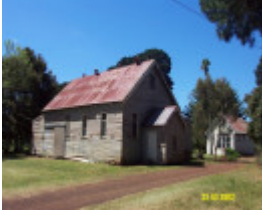
23541 Strathkellar Mechanics Institute 1904
