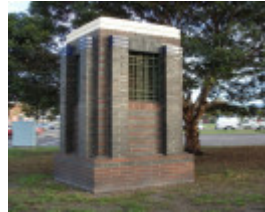
Underground toilet_West Melbourne_May 2007_brick ventilator
