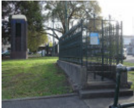
Underground toilet_West Melbourne_May 2007_general view
