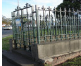
Underground toilet_West Melbourne_May 2007_railing detail
