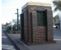
Underground toilet_Carlton_April 2007_ventilator shaft
