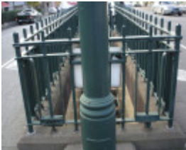
Underground toilet_Carlton_April 2007_railing detail
