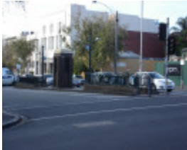
Underground toilet_Carlton_April 2007_view from NW
