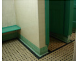
Underground toilet_Carlton_April 2007_interior of ladies'
