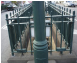
Underground toilet_Carlton_April 2007_railing detail
