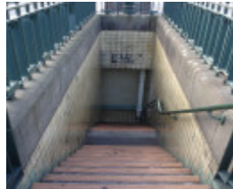
Underground toilet_Carlton_April 2007_ladies' stair
