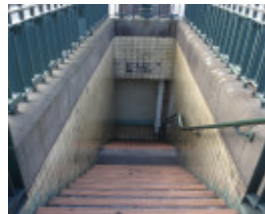
Underground toilet_Carlton_April 2007_ladies' stair
