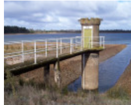
Stony Creek Outlet tower no. 3
