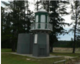
Stony Creek Outlet tower
