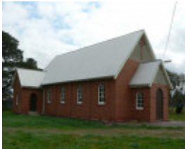
St Mary's Catholic Church, Midland Highway, Lethbridge
