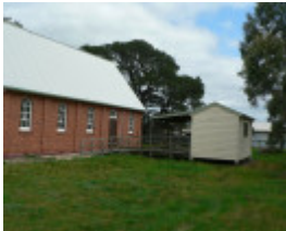
St Mary's Catholic Church, Midland Highway, Lethbridge
