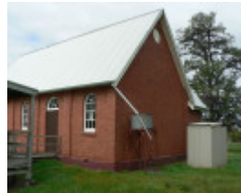
St Mary's Catholic Church, Midland Highway, Lethbridge
