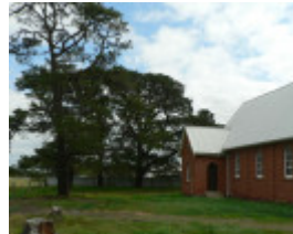
St Mary's Catholic Church, Midland Highway, Lethbridge
