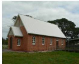
St Mary's Catholic Church, Midland Highway, Lethbridge
