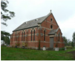
Former Presbyterian Church, Linton
