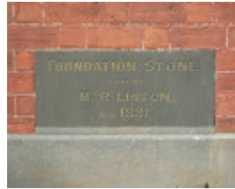
Former Presbyterian Church, Linton
