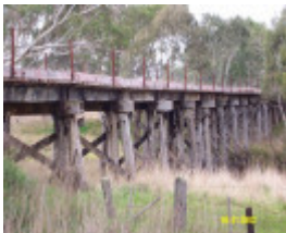
23621 Railway Trestle Bridge Wannon from W 1331
