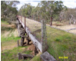
23621 Railway Trestle Bridge Wannon 1336
