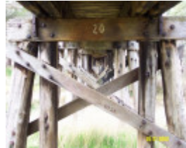
23621 Railway Trestle Bridge Wannon 1333
