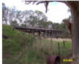
23621 Railway Trestle Bridge Wannon from W 1330
