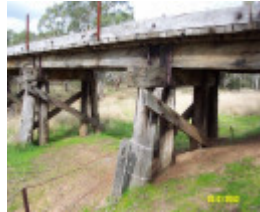
23621 Railway Trestle Bridge Wannon 1335
