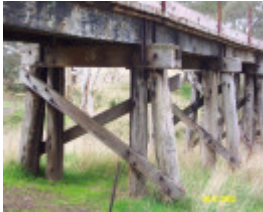
23621 Railway Trestle Bridge Wannon 1332
