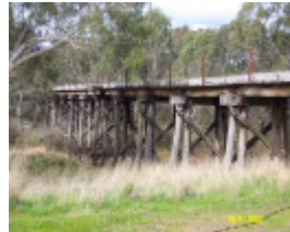
23621 Railway Trestle Bridge Wannon from E 1334
