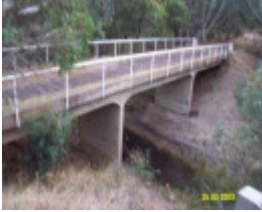
23628 Copy of 4471 Former Wannon Road Bridge Dunkeld
