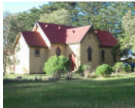
St Joseph's Catholic Complex, Meredith, Church from north-west
