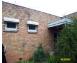
23643 Eaton Park Glenthompson front door 1222
