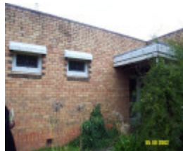
23643 Eaton Park Glenthompson front door 1222
