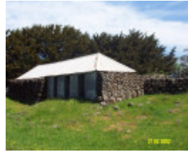
23644 Mirtschin Homestead complex cowshed 1855
