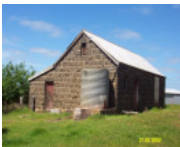
23644 Mirtschin Homestead complex stable 1851
