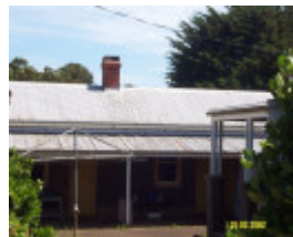
23644 Mirtschin Homestead complex service wing 1849
