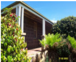
23644 Mirtschin Homestead complex verandah 1852
