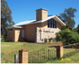
23656 St Mark s Anglican Church Cavendish 2077
