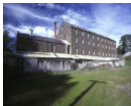
1 andersons mill complex off alice street smeaton front view jul1987
