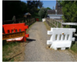
bridge with barriers.jpg
