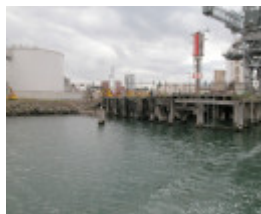
ICIANZ Chemical Factory Wharf Maribyrnong May 2003 003
