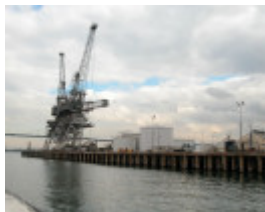
ICIANZ Chemical Factory Wharf Maribyrnong May 2003 004
