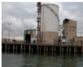
ICIANZ Chemical Factory Wharf Maribyrnong May 2003 001
