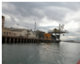
ICIANZ Chemical Factory Wharf Maribyrnong May 2003 002
