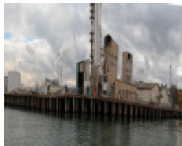
ICIANZ Chemical Factory Wharf Maribyrnong May 2003 005
