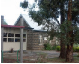
Shelford Primary School
