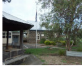
Shelford Primary School
