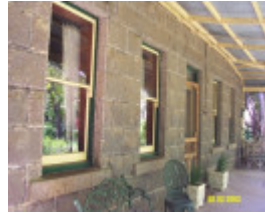
23745 Sylvan Grove Croxton East facade 1766
