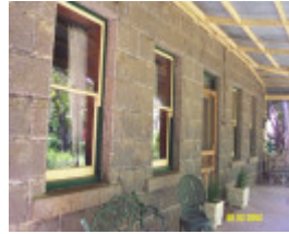
23745 Sylvan Grove Croxton East facade 1766
