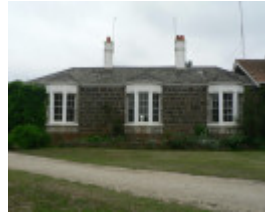
Woolbrook Homestead south elevation
