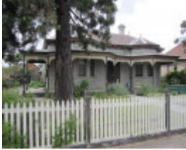
House 262 Ascot Vale Road
