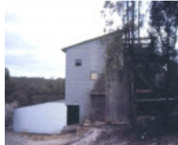
h01879 wattle gully gold mine fryerstown road chewton battery house she project 2003
