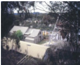
h01879 wattle gully gold mine fryerstown road chewton engine house she project 2003
