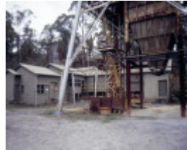
h01879 1 wattle gully gold mine fryerstown road chewton poppet head she project 2003
