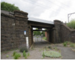
Bloomfield Road Rail Overbridge.JPG
