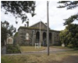
PORT FAIRY COURT HOUSE SOHE 2008
