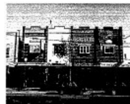
23893 Shops with residence
