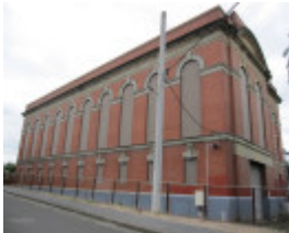
Newmarket Railway Substation.JPG
