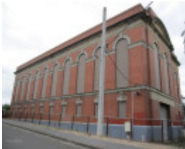
Newmarket Railway Substation.JPG
